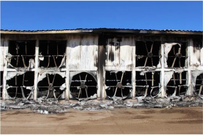
A photo from the Texas State Fire Marshal's Office report shows fans in the cross-ventilation barn melted from the fire. STATE FIRE MARSHAL'S OFFICE/ TEXAS DEPARTMENT OF BUSINESS
